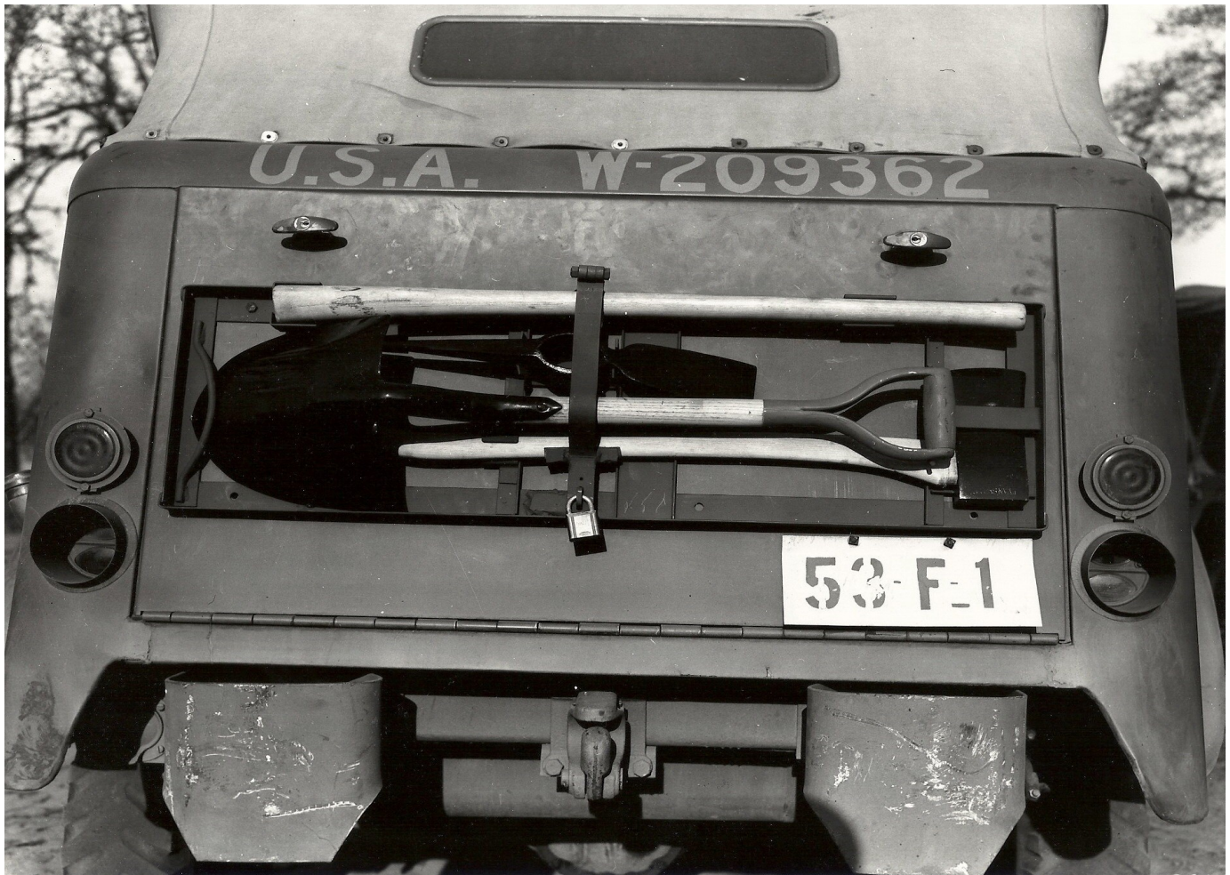
Dodge 1/2 ton Command Car tailgate showing pioneer rack and tools.
