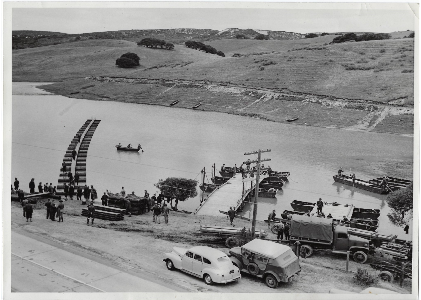
Couple of interesting photos. Top: USN Base during a rainstorm lots of early rare vehicles far left towing a Jeep is a M-3H-4 1.5 ton wrecker. Far right heading toward the photographer is a Dodge WC 1/2 ton panel truck. USMC Bottom: Shows an Army Engineer group Early WW2 practicing bridging. Acme News SF.
