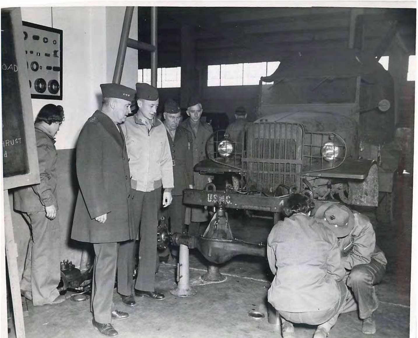
1944- Lt. Gen. A.A. Vandergrift with Maj. Gen. Henry Larsen during inspection tour of the Marine Corps training base at Camp Lejeune. Here they watch as members of the Marine Corps Women's Reserve studying at the Motor Transport School repair a truck axle. (The truck being repaired is an International M-2-4 1 ton Ed.)
